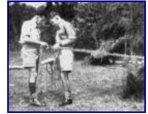
Joining the strands prior to lay up.
